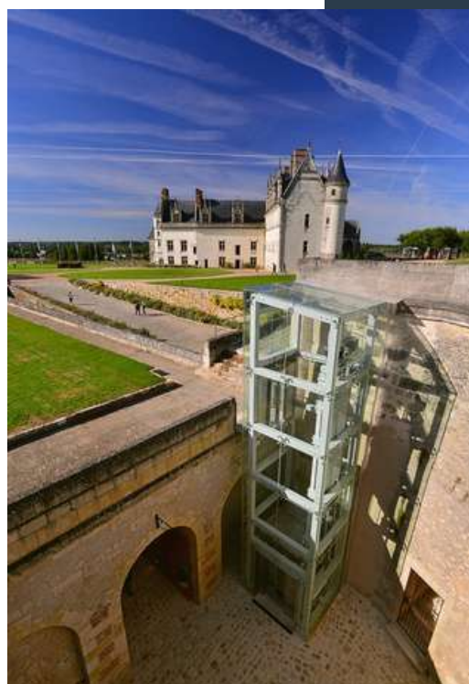
Elevator leading from the ticket/shop level to the toilets (1st level) and to the gardens/lodgings (2nd level).
